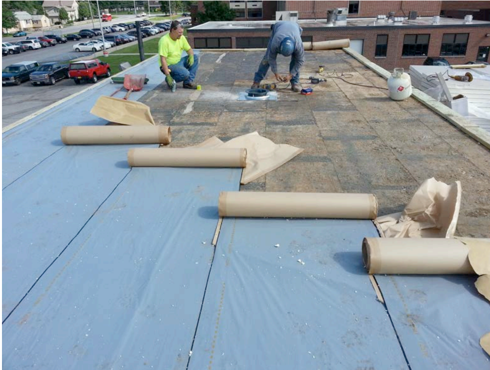
Buildings & Grounds Upper Roof Deck (Vapor Barrier & Roof Drain Install)
