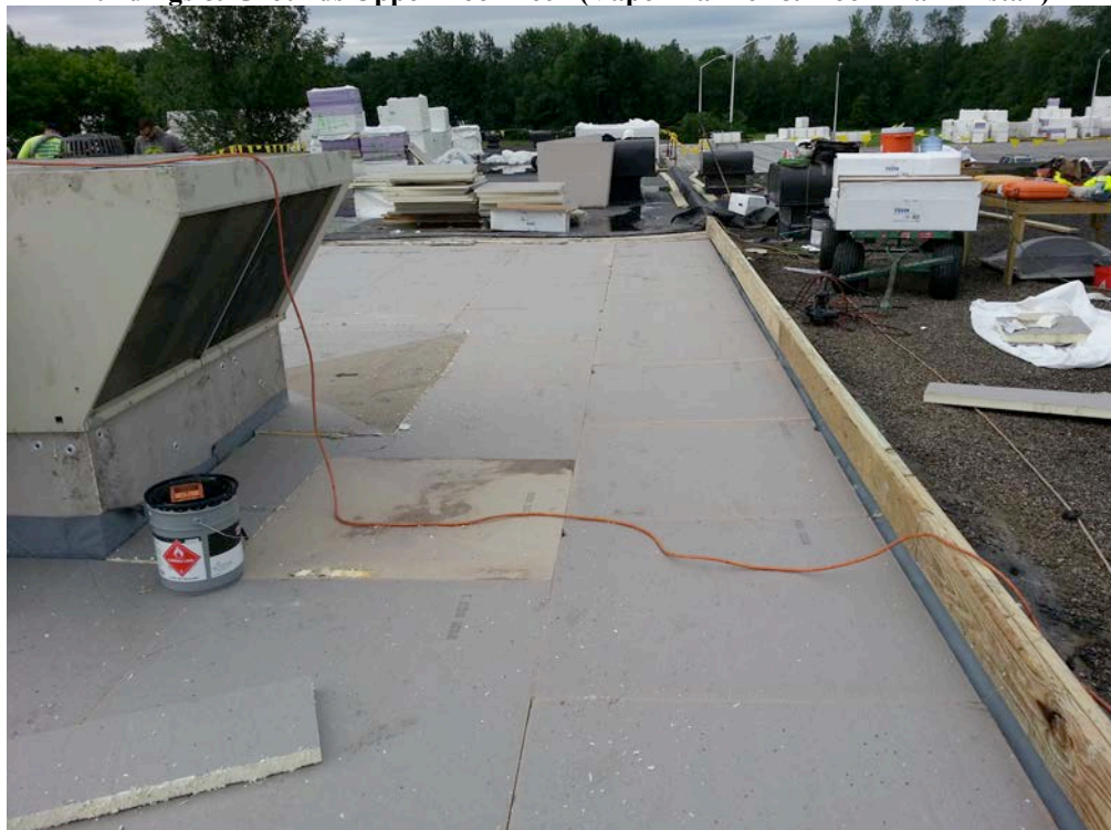
Ledgeview Elementary Roof – Start of New Roofing System Installation
